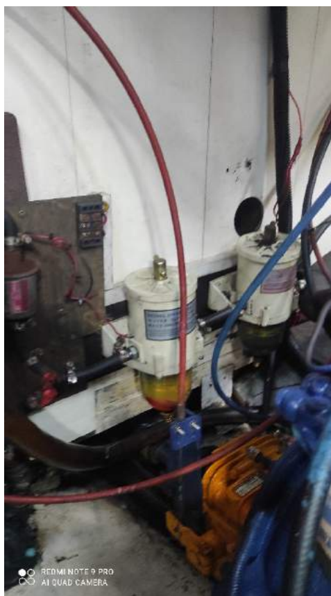
67_dieselfilter_electric_transfer_pump
